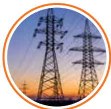
Modernize the Electrical Grid
