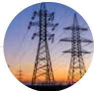
Modernize the Electrical Grid
